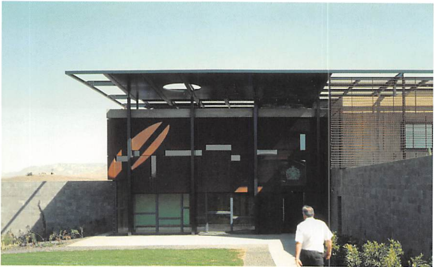
Consular and Visa Section; the slot windows are of coloured glass within 'weathering' steel panels. The wall to the right is of habash volcanic stone.
