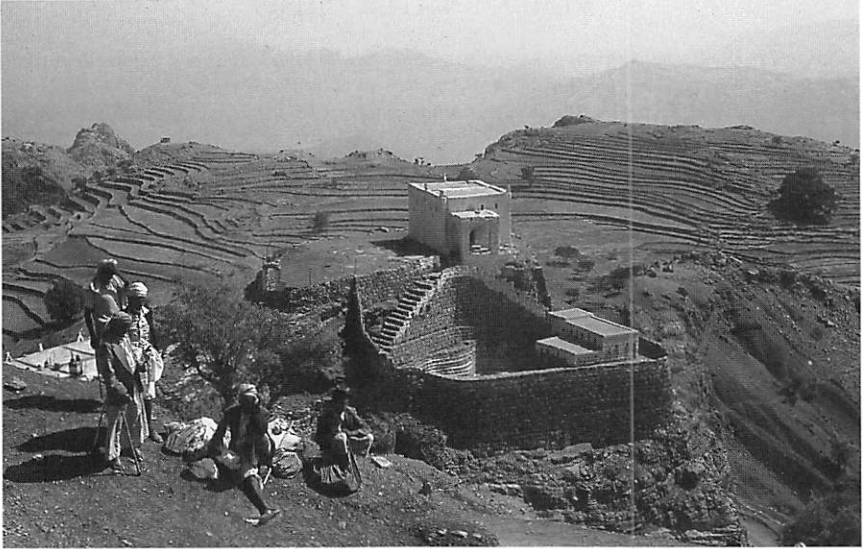
Cistern at Kuhlan, a casualty of road construction.
