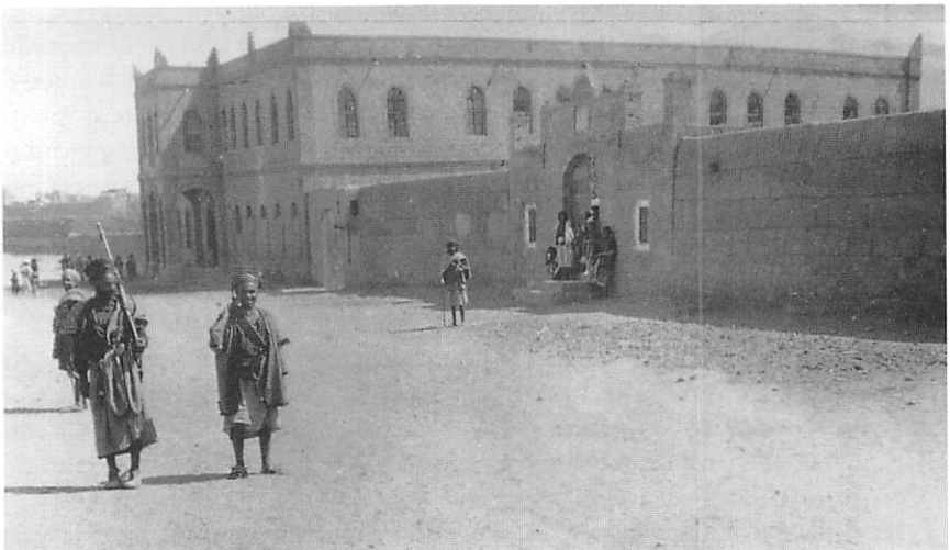
The Guest-house overlooking Maidan al-Shararah (Tahrir Square), which is now the Military Museum. In the foreground two members of the Mission's permanent guard.
